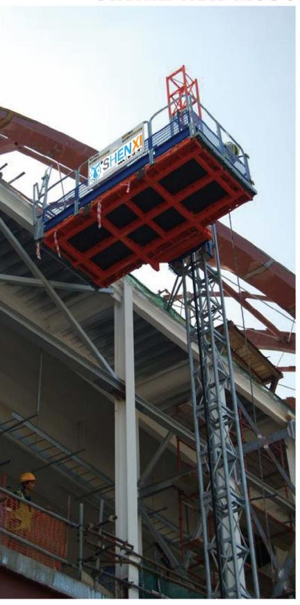
SHENXI's Modular System STP and SMH were designed to bring versatility and efficiency to the industry. With relatively few components, it can be configured to create various work platforms, transport platforms, or a combination of both.
